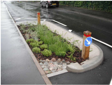
Plate 1 – Roadside SuDS recently installed by BCC in Southmead (note the plants have not matured)
